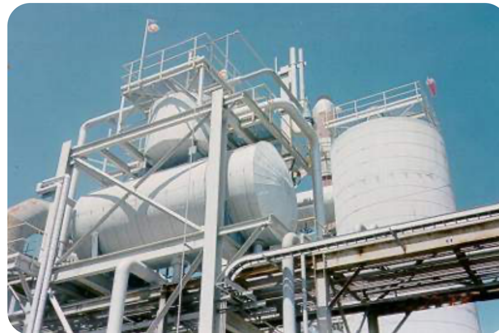
Vertical Tray Deaerator Capacity: 1,000,000 lb/hr Best for Refineries and Utility Thermal Plants
